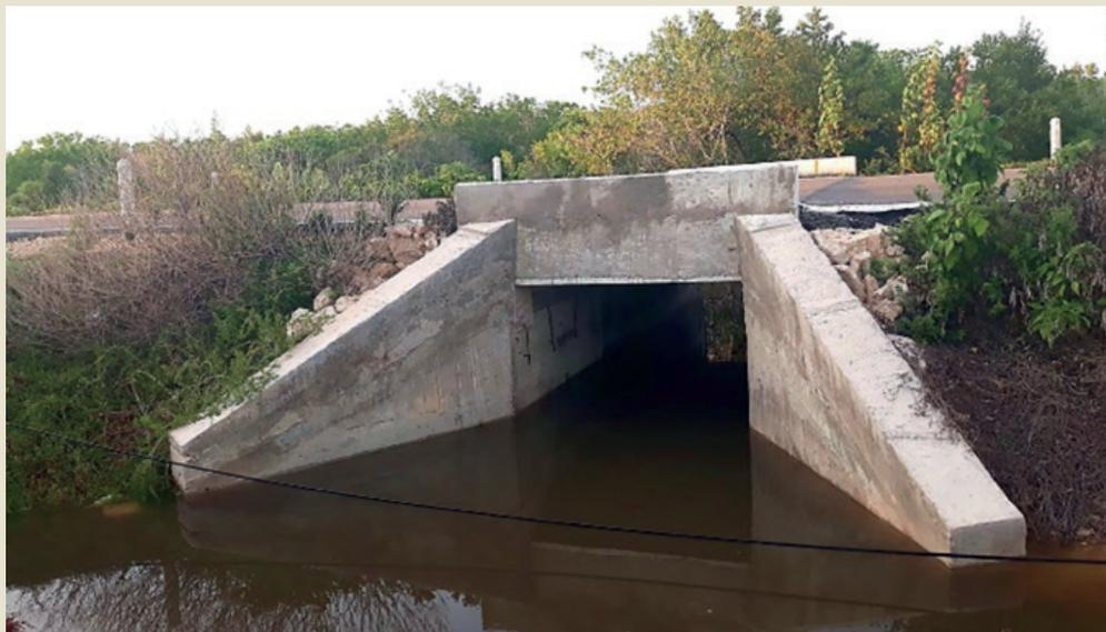
Desilted culvert with an inverted “Y” shape
