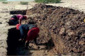
The excavation can be carried out in layers, at least 1 m in depth or where the mother rock allows. It is important that it must resemble the natural configuration of canals.
